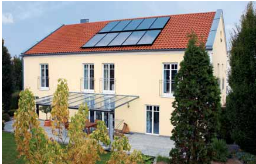
Vitosol 200-FM Two-family house, Geisenfeld
